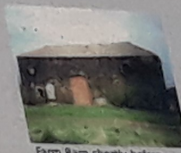
Farm Barn shortly before demolition in 1995
